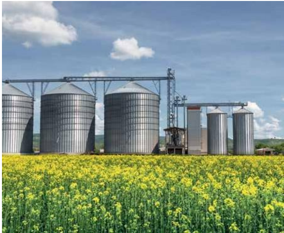
Microorganisms circulating in the air make food perishable – especially in tanks and silos.
